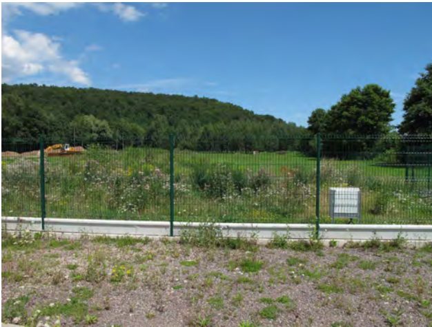
Station S36, site en construction, ZA Muhlbach-sur-Bruche, 31/07/2010
